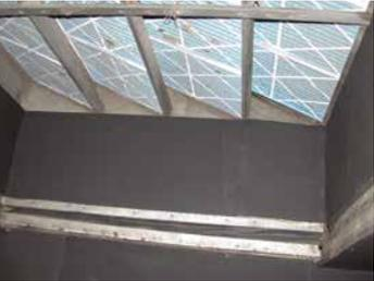
In all cases, Waterbury Schools opted to use AP Armaflex closed cell elastomeric duct liner to replace the open cell liner in the air handling units. The decision was based on the strong recommendation of Jim Choquette, who cited numerous reasons why his company preferred to work with closed cell Armaflex material.
