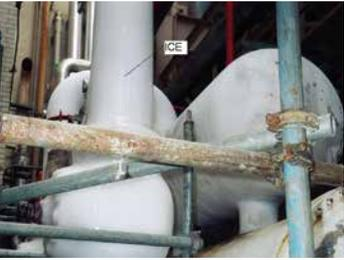
The result was a clean-looking, reliable insulation that should last the plant a number of years. While Bob Mask of Insulation Specialties, the installation contractor admits that cutting the 2-inch foam required a certain amount of precision, the final product was worth the effort.
