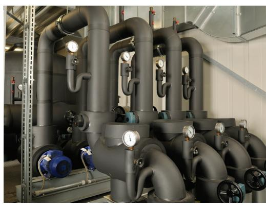
Armacell's newest innovation, ArmaFlex Ultra with FlameDefense<sup>™</sup> Technology, is the first elastomeric foam insulation Classified by UL to UL 723 at 25/50. This third-party certification proves our commitment to product safety and compliance. All AP/ArmaFlex-branded products are made with Microban<sup>®</sup> antimicrobial protection, are GREENGUARD Gold certified and now have Environmental Product Declarations (EPDs) to show our dedication to material transparency.
